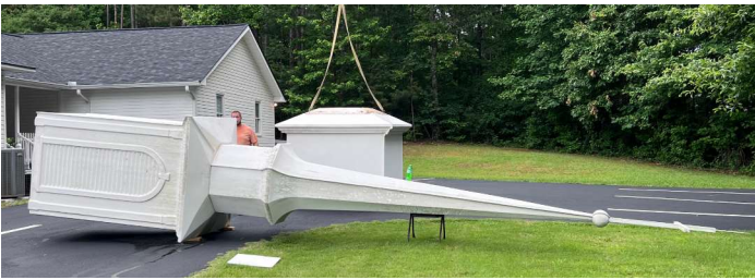
Lakeview had their church steeple removed, repaired and replaced.
